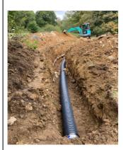
After further clearance work on the open leat, the entire system was connected for testing in early May and we are delighted to say that there is an excellent flow of water all the way from the spring to the point where the Forebay tank will be (just to the left of the access road near the Coach House). This provides filtration and control.
